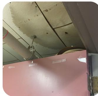
ABOVE L: The roof system at Connors is past its useful life, showing leaks.
